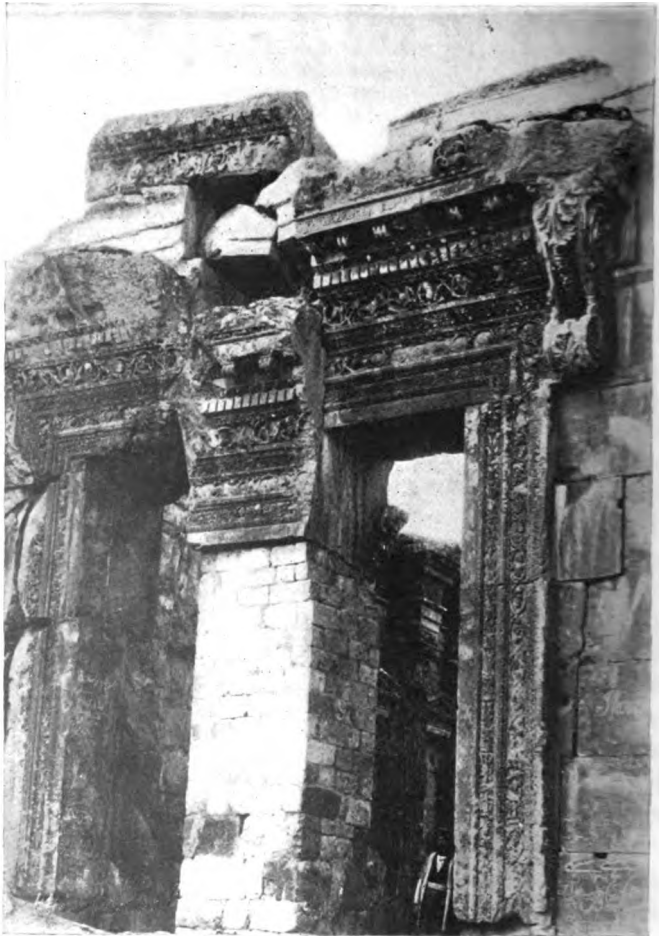
Roman Doorway at Baalbec.
